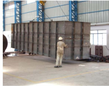
Fabrication & Assembly Facility at Hosur, Tamil Nadu
